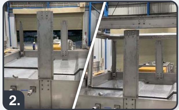
2. Install vertical support and frame in basin.
