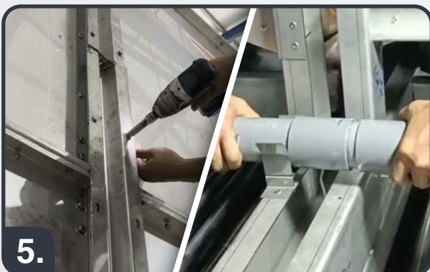
5. Install panel support on gap and spray branches inside the unit.
