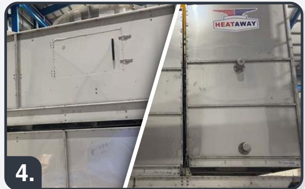
4. Mount both of fan sections to coil section and bring them to mount on basin section.
