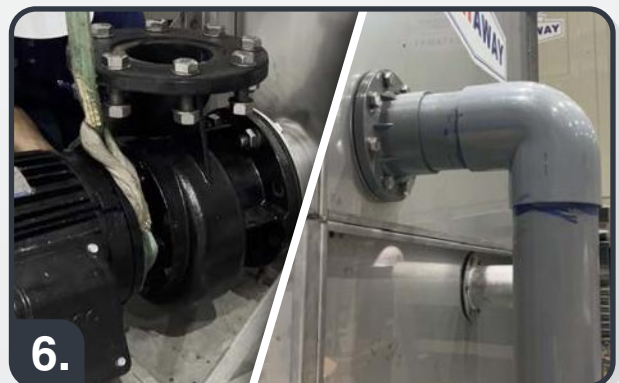
6. Mount water pump and water piping.
